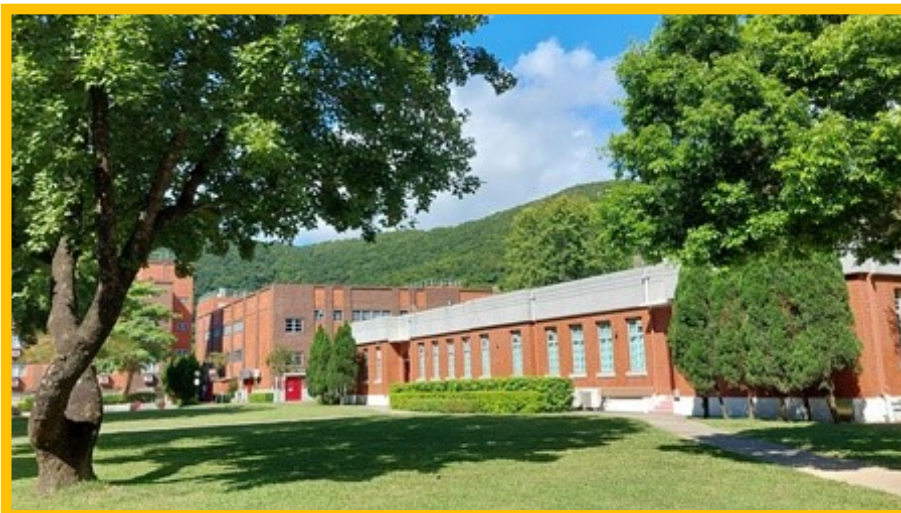
Reverse facade of Elder Chu Yue-Tat designed Sam Yuk Middle School (Clear Water Bay campus) historic, grade 2 listed, Art Deco style building with part of the HKAA building and part of the campus dormitory building on the left side
