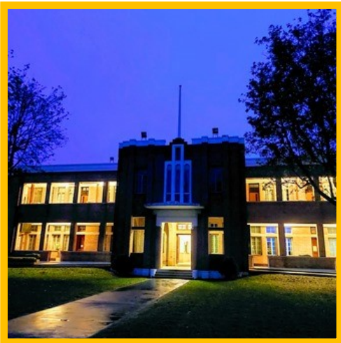
HKAC Administration’s historic, grade 2 listed, Art Deco style building designed by Elder Chu Yu-Tat (朱如達長老) in the 1930’s. Elder Chu had been a civil engineering student at Lingnan University.
