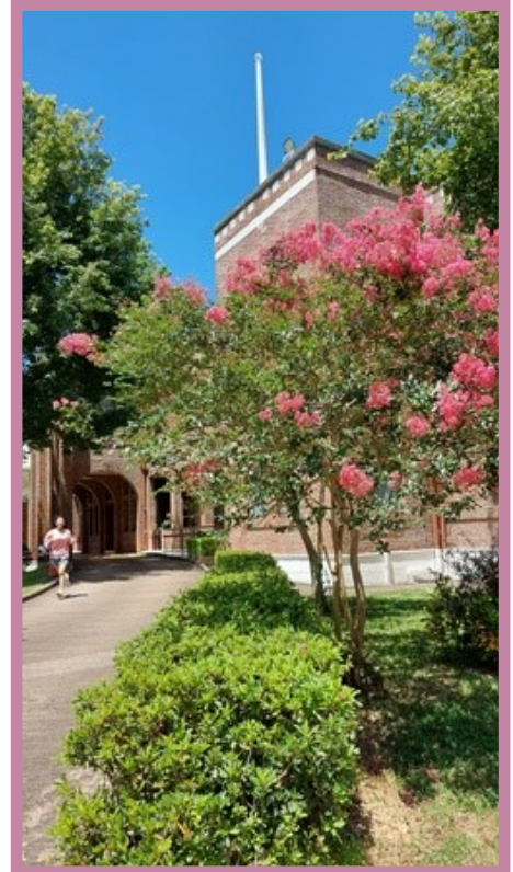
Diagonal front view of the HKAC, grade 2 listed, Administration building with a jogger who has emerged from the portico
